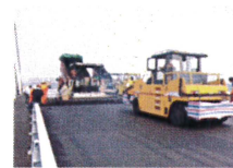
Paving of KT-BEP
